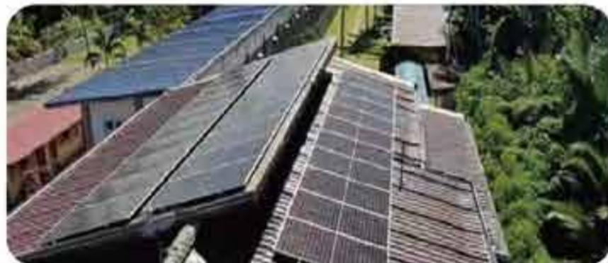
20KW Hy-Grid Solar System In Indonesia
